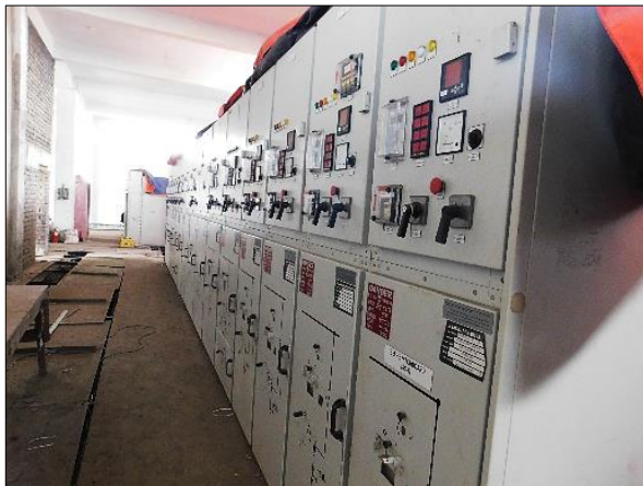
Indoor Substation Switchgear Room with 33 kV and 6.6 kV Panels
